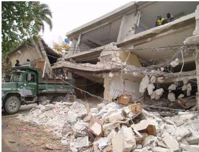
(Earthquake destruction at Trinity School in Port-au-Prince)
